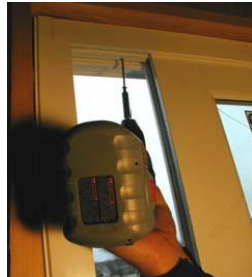
Screws placed just above the door in the header, eliminating upward motion.
