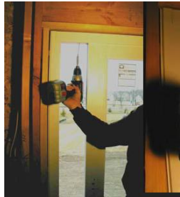
Screws placed just above the door in the header, eliminating upward motion.
